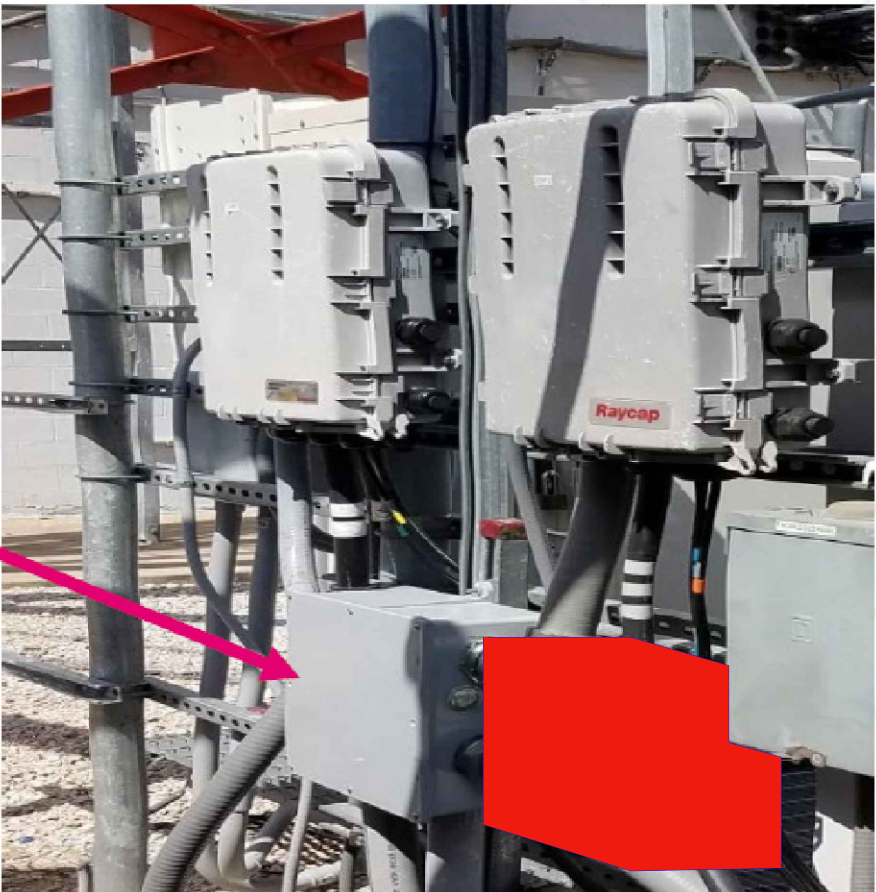
DALLAS SOA INSTALL
