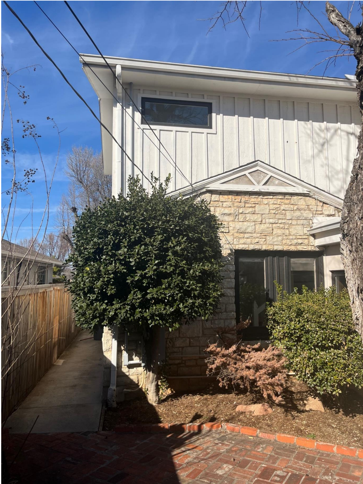
West Side Facing North
