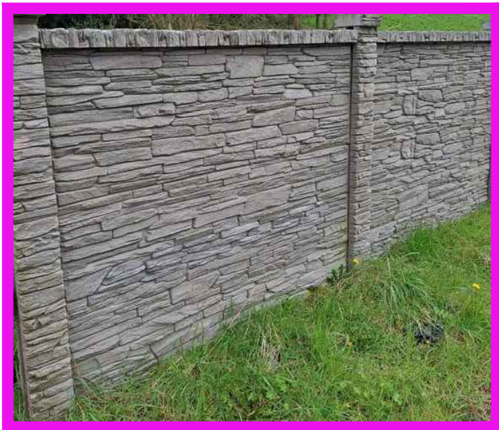
FENCE 1C DESCRIPTION: 8' TALL MODULAR PRECAST STONE WALL COLOR MATCHED TO EXISTING STONE
