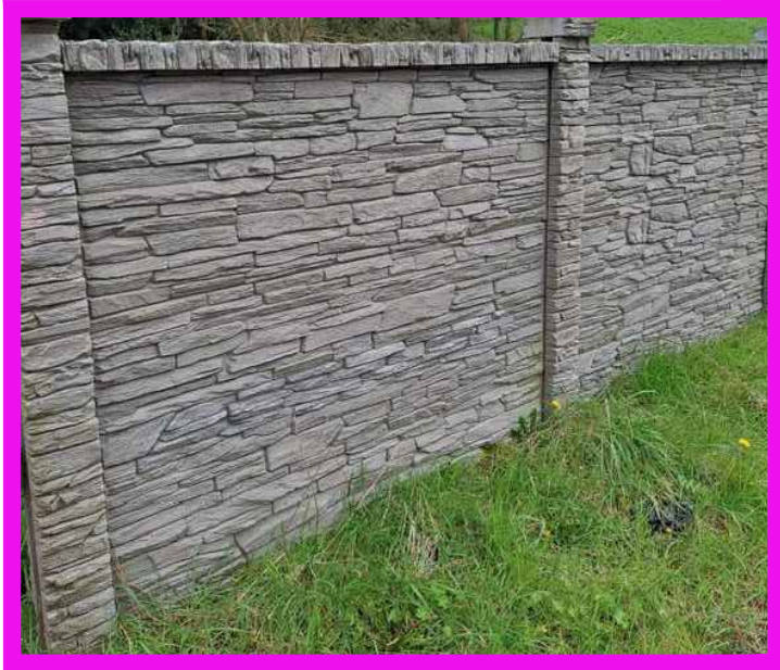
FENCE 2C DESCRIPTION: 8' TALL MODULAR PRECAST STONE WALL COLOR MATCHED TO EXISTING STONE
