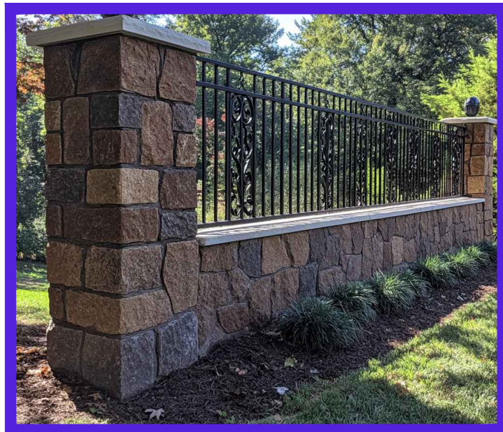
FENCE 2A DESCRIPTION: 2' TALL MASONRY STONE PONY WALL 6' WROUGHT IRON FENCE ON TOP WITH ACCENT COLUMNS
