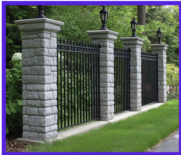
FENCE 3A DESCRIPTION: 8' WROUGHT IRON FENCE WITH ACCENT COLUMNS. STONE COLOR TO MATCH EXISTING
