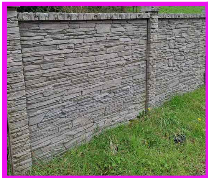
FENCE 3C DESCRIPTION: 8' TALL MODULAR PRECAST STONE WALL COLOR MATCHED TO EXISTING STONE
