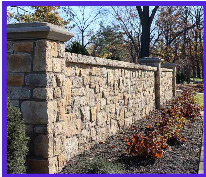
FENCE 1A DESCRIPTION: 8' TALL MASONRY STONE WALL WITH ACCENT COLUMNS. STONE COLOR TO MATCH EXISTING
