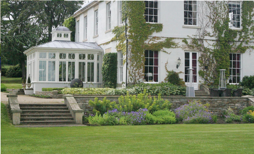
Insp for Orangery roof
