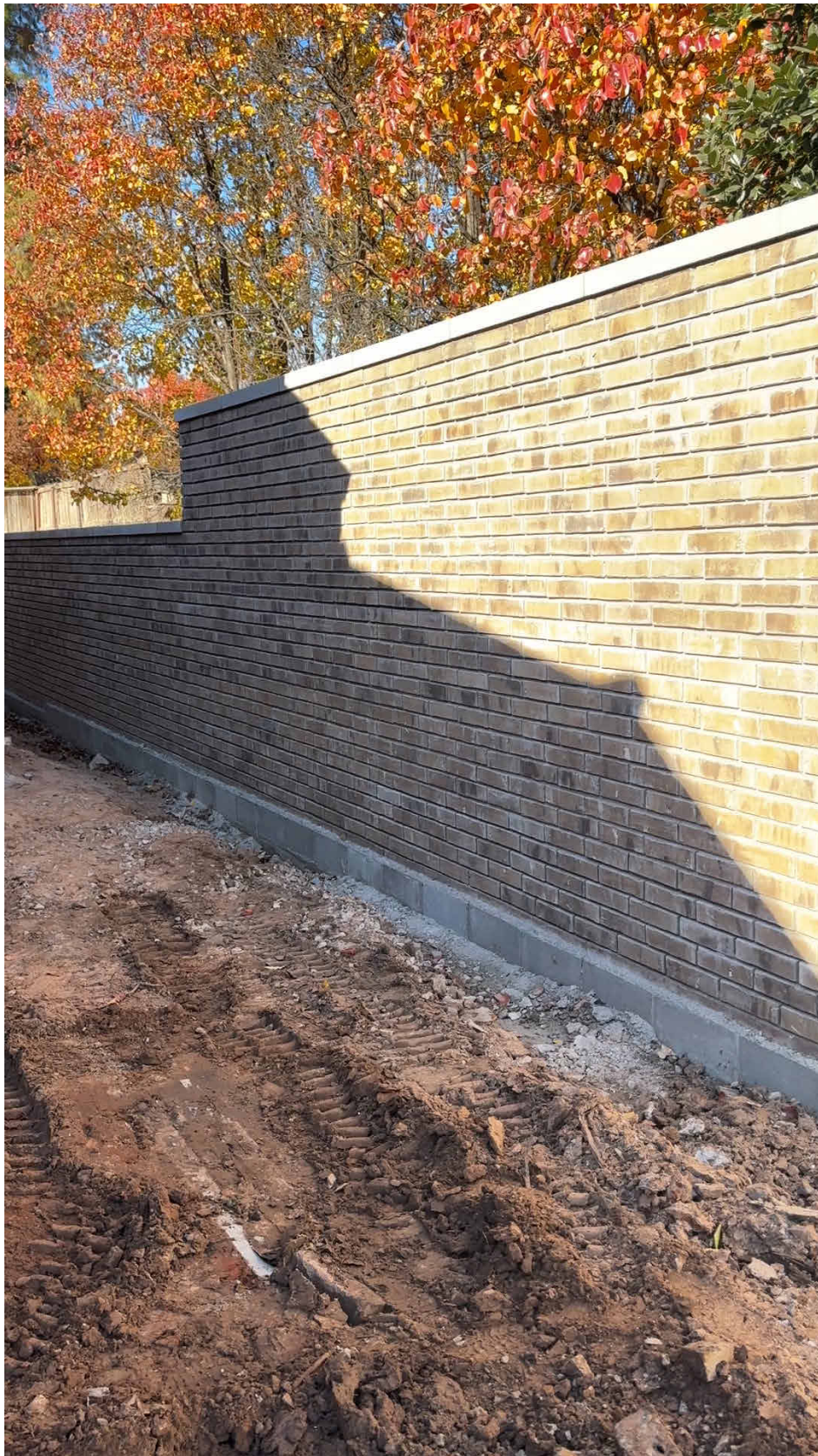
BELOW: RE-BUILT RETAINING WALL
