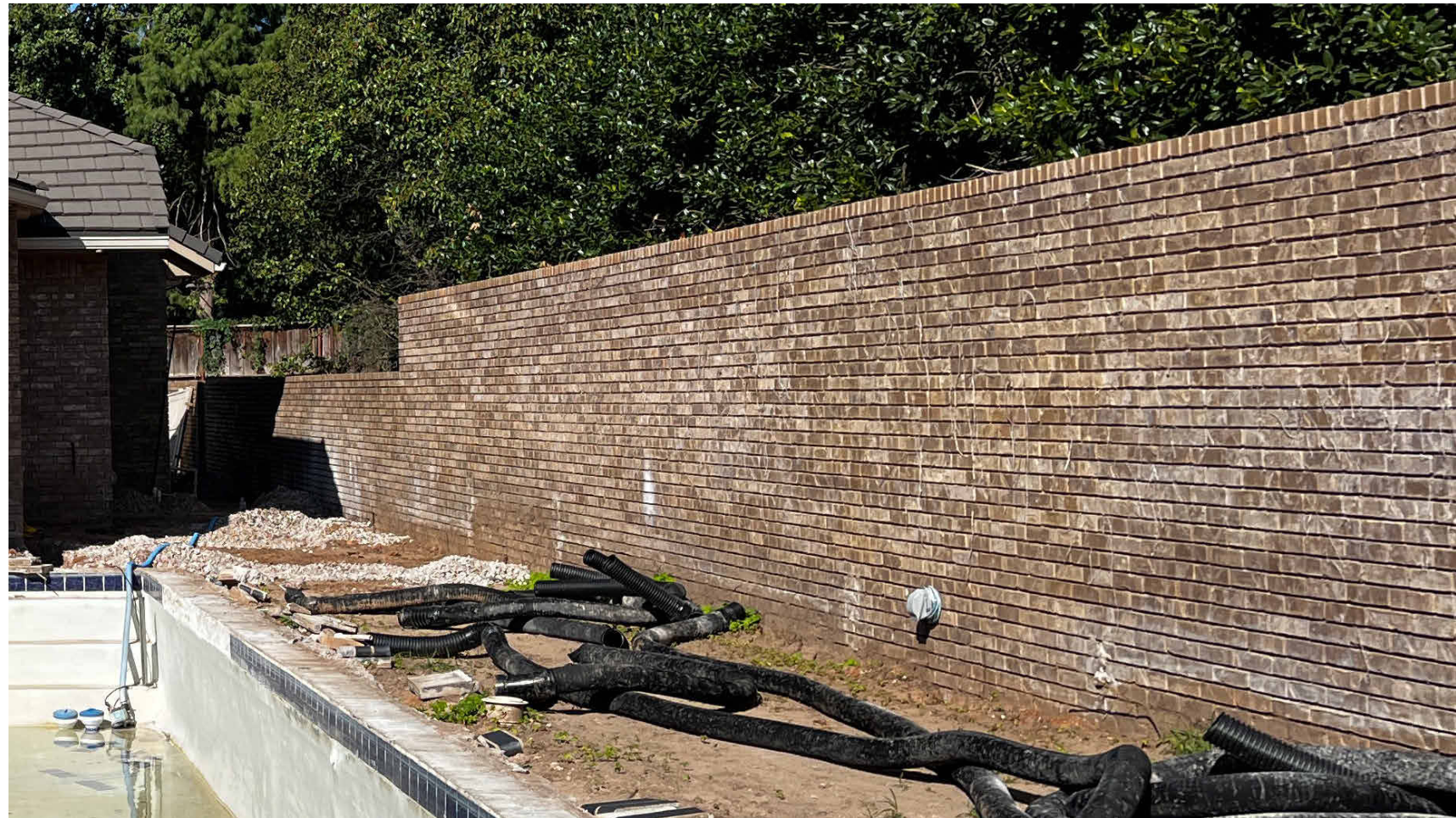
ABOVE: RETAINING WALL PRIOR TO COLLAPSE.
