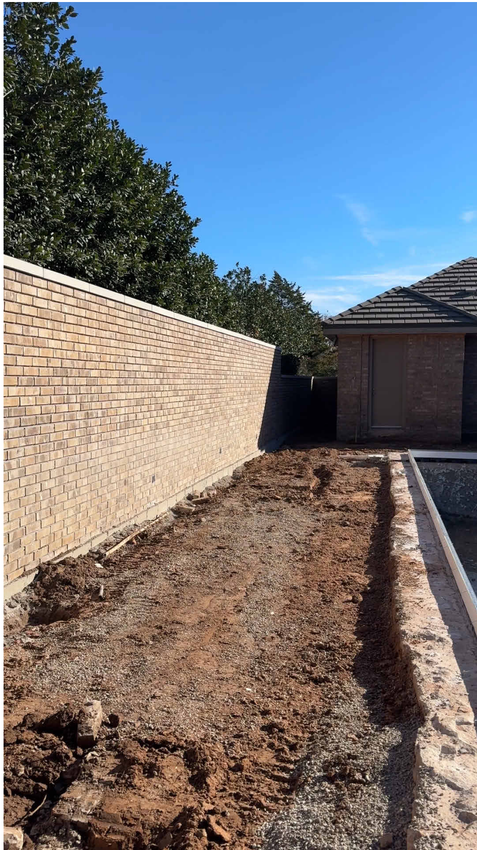
BELOW: RE-BUILT RETAINING WALL
